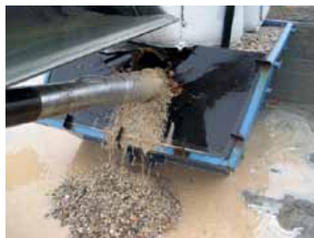
▲ Figure 3: After drilling through biological cemented gravel (left) the borehole remained stable (right).
