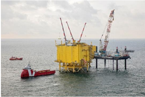
Presently involved in hook up and commissioning work (lower margin)
