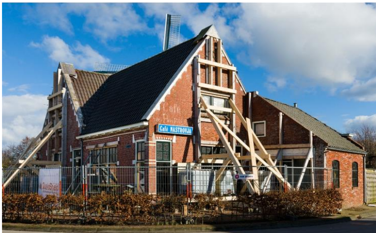
Figure 1: Building in Groningen strengthened with wooden frames
